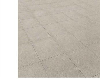
11 - Marshalls Perfecta Smooth Ground Flag Paving with Yorkstone aggregate (or similar) to main terrace area replacing existing patchwork of paving
