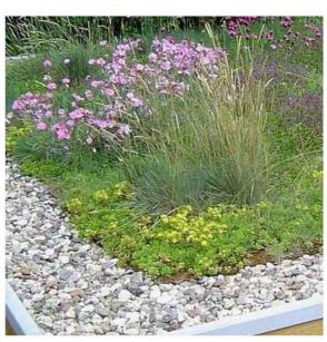
**06** - Sedum roof with gravel perimeter drainage and internal drainage
