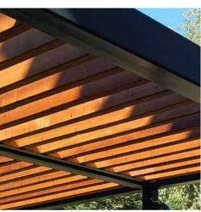
**07** - vertical timber slat canopy set into dark grey metal frame to match glazing
